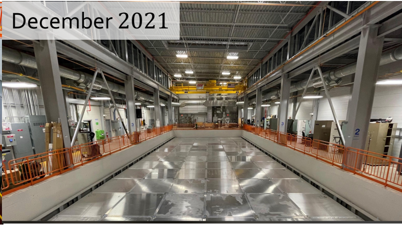
Completion of CRT installation
